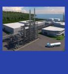
Production of E-Methanol based on green hydrogen and C02 captured from industry. Unit with a production capacity of **70 kt**. Project does not include the production of green hydrogen. Final product mainly used in the chemical industry and as a synthetic fuel
